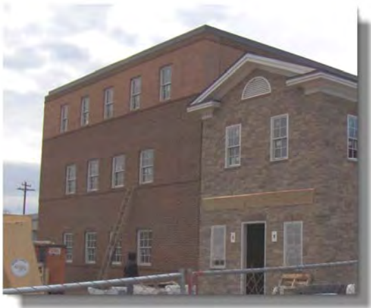
Nelson Clinic in final stages of construction
